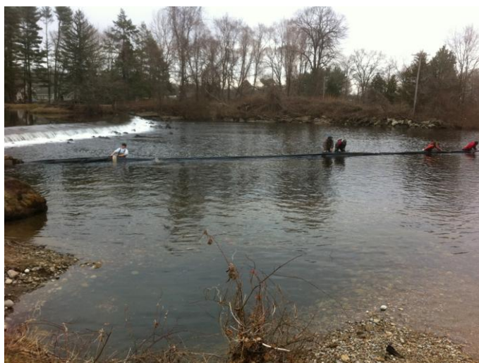
CTDEP and TNC crews work to install the fish guidance boom below the Wood Dam Fishway (out of the photo, to the left). The boom is connected to the fishway to the left and a big boulder to the right to help guide fish to the fishway, particularly during high tide.
