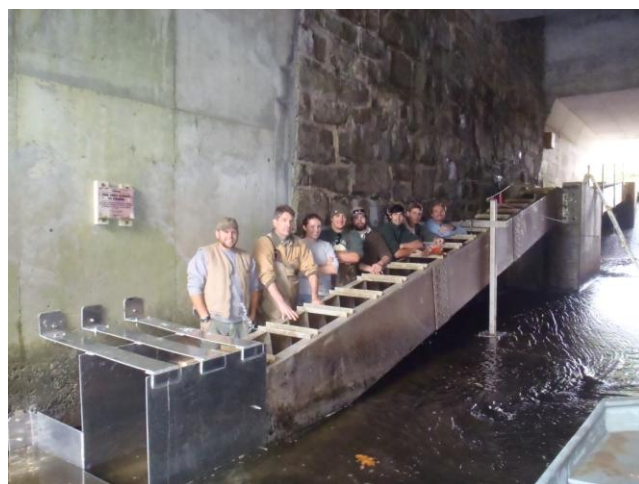
The repaired Trading Cove Brook Fishway with a new entrance to the left of Dave and a new intermediate support to the right of me. L to R: Dave Ellis, Tim Wildman, Jessica Bell(s), Jeremy Grous(s), Ryan Mowrey(s), Aaron Grade(s), Bruce Williams, Steve Gephard. [s= 2010 seasonal employees]
